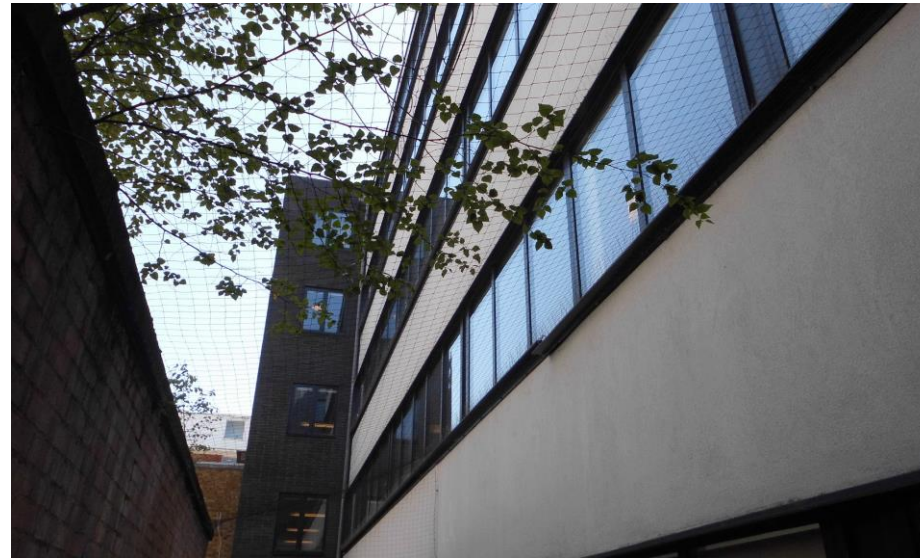
Existing north façade – showing typical window (none opening)
