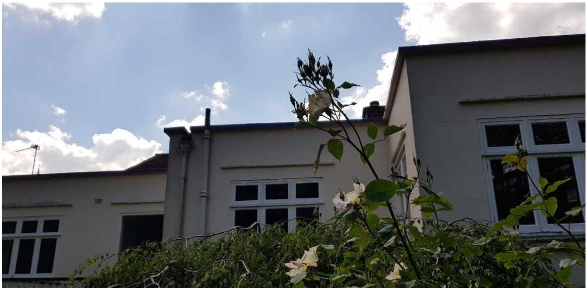
Figure 17: Rear elevation showing the identical proportions of the three upper floor windows and the tile details above the openings
