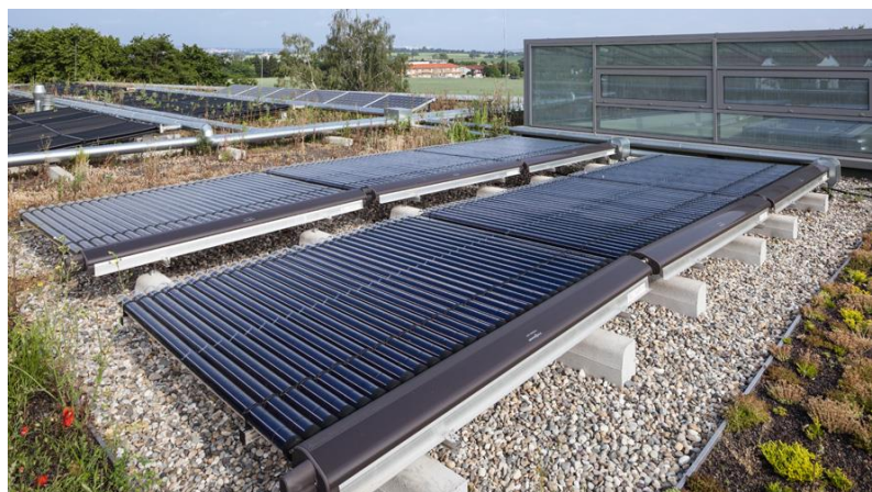
Vacuum tube Solar Thermal Collectors
