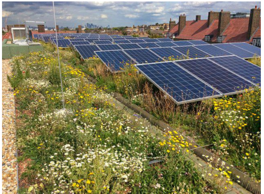
PV Panels integrated with green roofs
