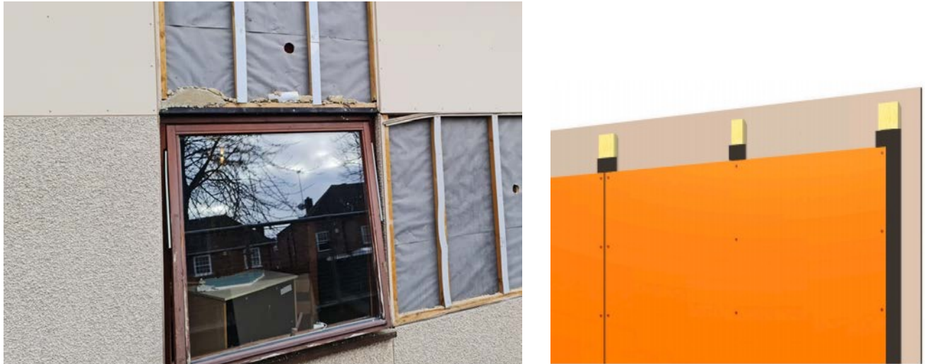
Picture 5 - Existing elevation survey and Steni fixing system diagram
