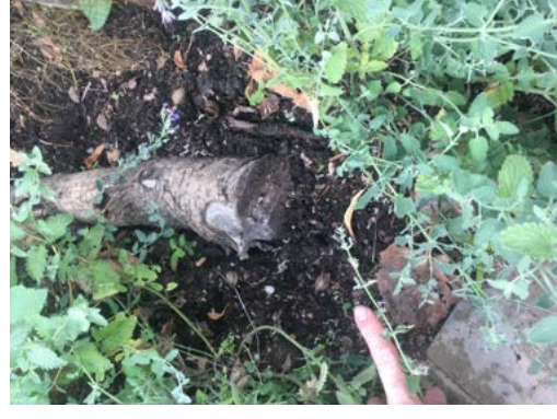
Severed anchorage root (150mm diameter) to south of main stem
