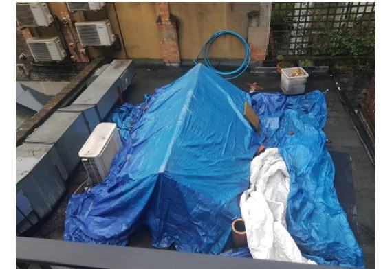
Figure 25 – Temporary measures to prevent further water ingress at rear roof
