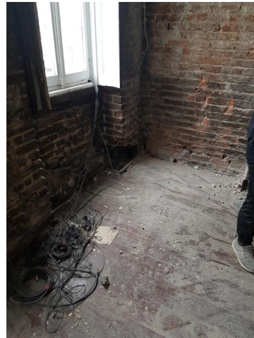
Figure 4 – Cracking of L01 South Party Wall – Note undermined pier
