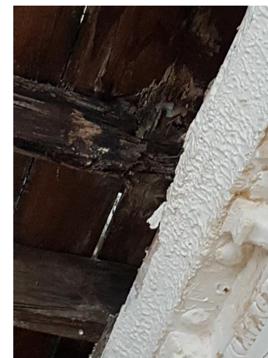
Figure 21 – Close up L02 timber joist with full loss of section
