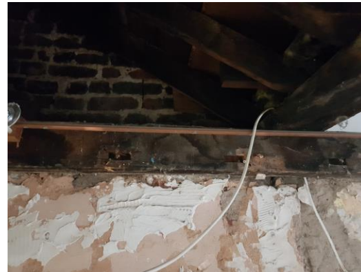
Figure 23 – Water stained timber likely due to water ingress at roof level
