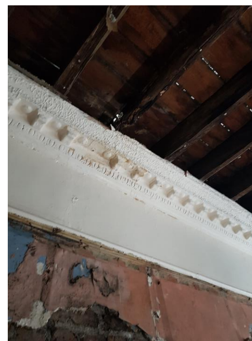
Figure 20 – L02 timber joist with full loss of section
