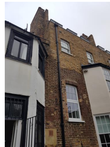
Figure 12 – Rear Facade – Note bulging brickwork at eave of bay window
