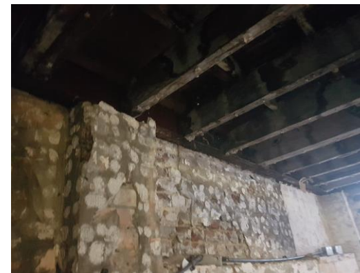
Figure 26 – Rear building ground floor joists from below, note water staining
