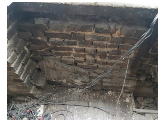
Figure 7 – Poor bonding of front façade brickwork at L01
