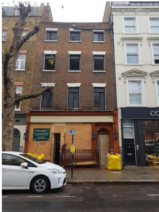
Figure 3 – Front Facade – Note drop in brick coursing above centre window
