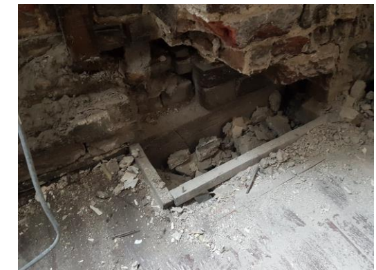
Figure 8 – Undermined pier and timber beam at L01 South Party Wall
