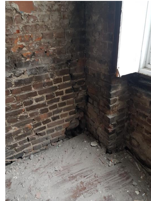
Figure 5 – Cracking of L01 North Party Wall
