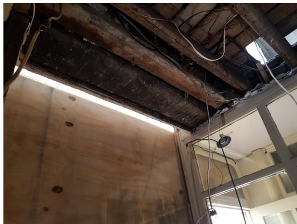
Figure 9 – L01 front façade timber beam from underside
