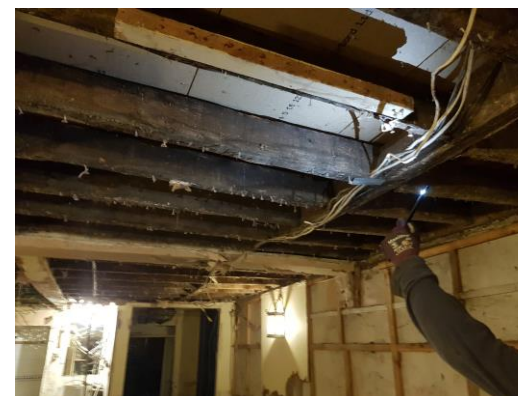
Figure 18 – Ground floor joists dropped – note gap between floor boards and joists
