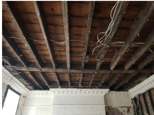
Figure 22 – Third floor bressummer from underside – note visible bowing
