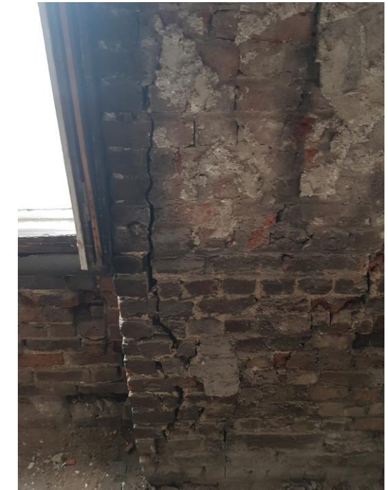
Figure 6 – Cracking of L01 centre pier
