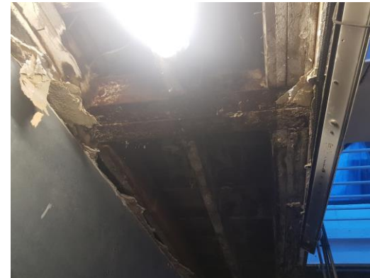
Figure 24 – Corroded beams at rear roof adjacent to Party Wall
