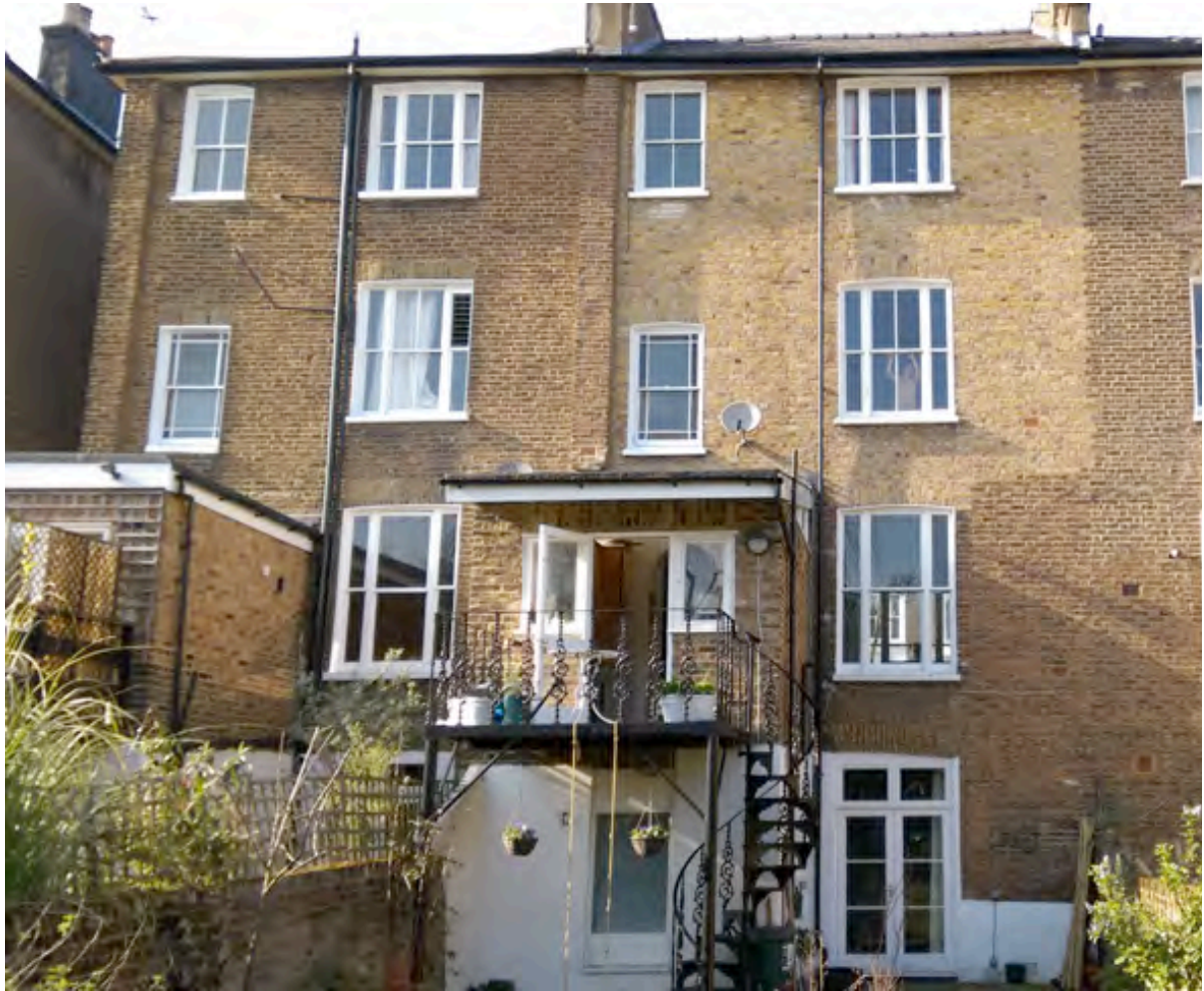
overall view of rear garden elevation
