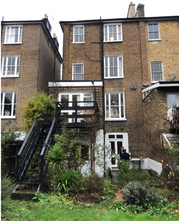
side of no. 41 closet wing w/ high level windows
