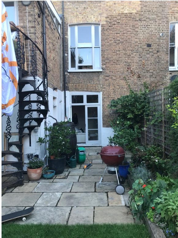
view of closet wing w/ high-level windows
