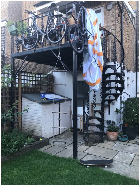
existing balcony w/ spiral stair
