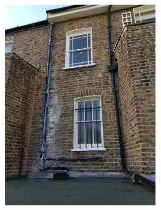
The existing window will be replaced with a timber framed door with Georgian bar glazing to match the character of the other windows.
