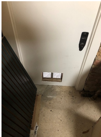
Figure 2: Existing ventilation grate in lightwell door
