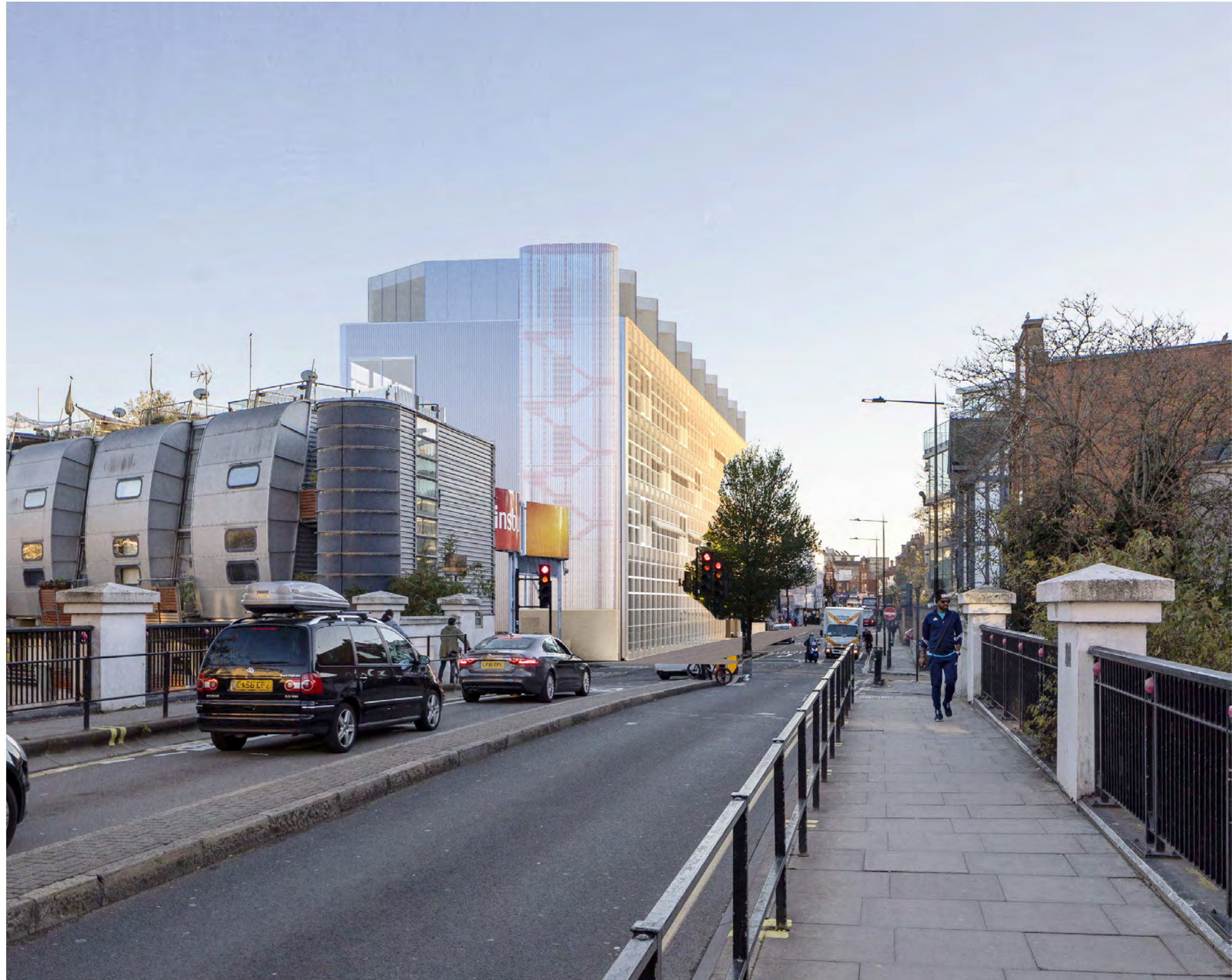
Work in Progress View from North West
