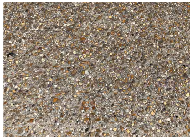
Refurbished existing exposed aggregate concrete roadways
