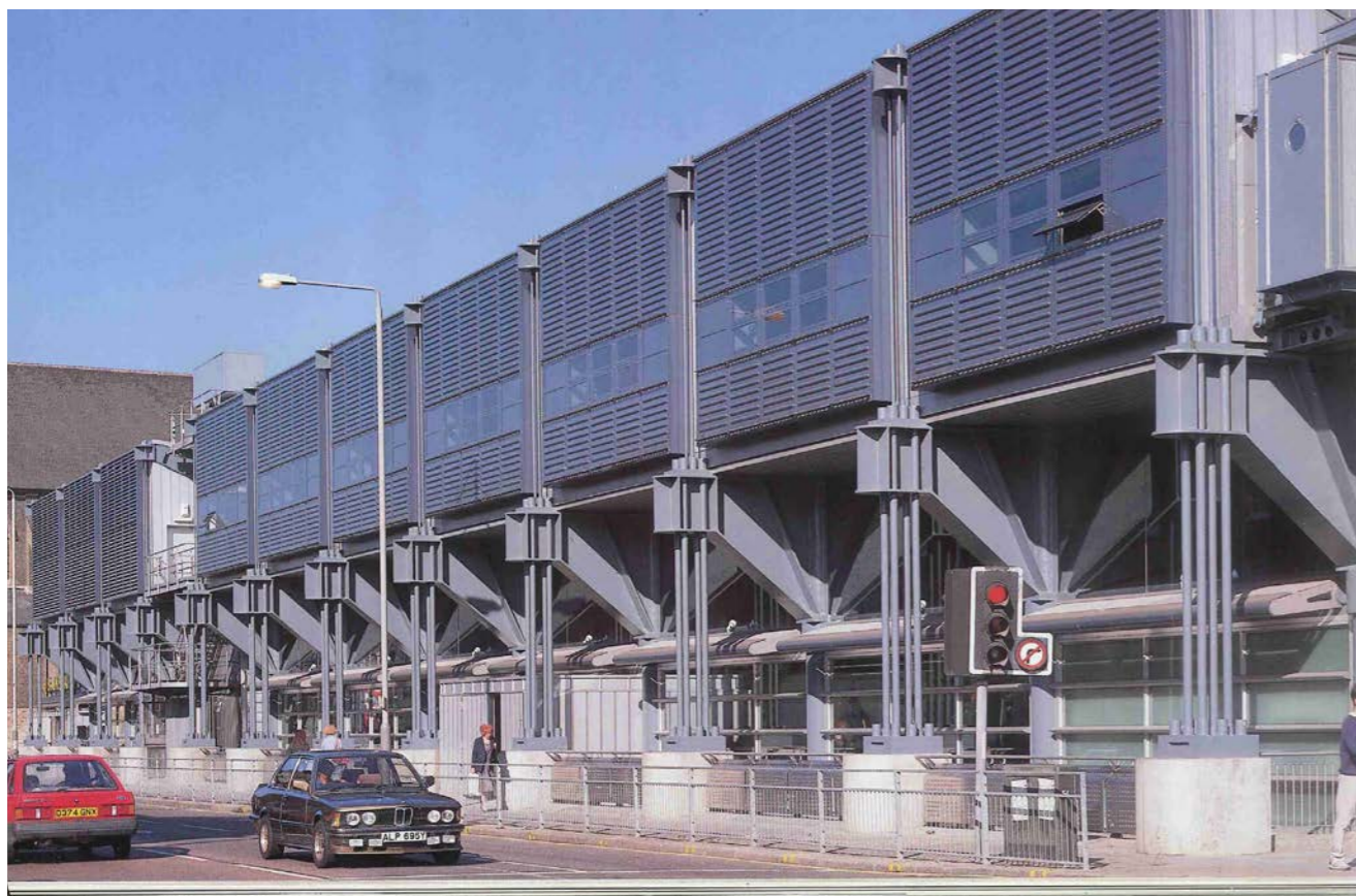
Figure 28. 1989: Sainsbury's by N. Grimshaw shortly after opening (Architectural Review, October 1989)
