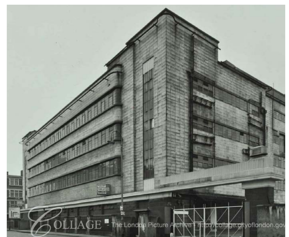
Figure 19. 1973: Aerated Bread Company, nos 133-147 Camden Street (LMA).
