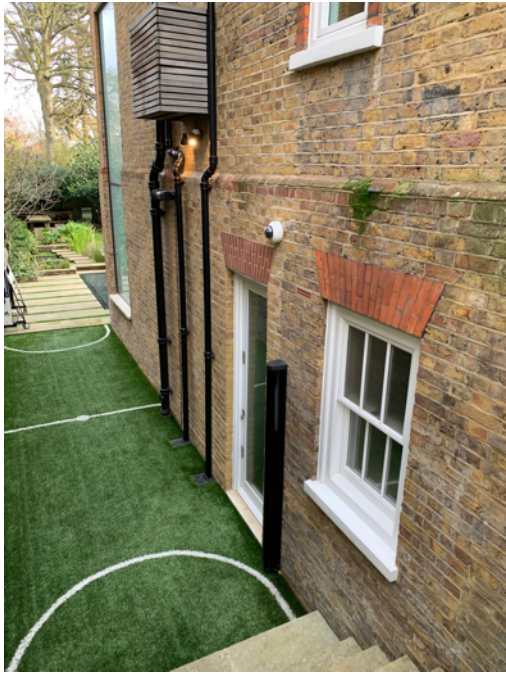
5 Side passage at 3 Holford Road
