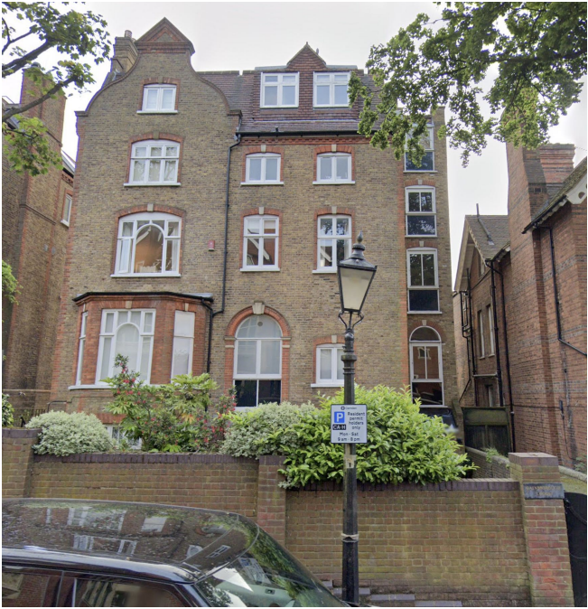
3 2 Holford Road, from the highway
