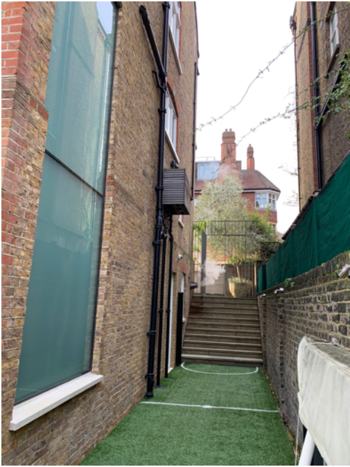
6 Side passage at 3 Holford Road
