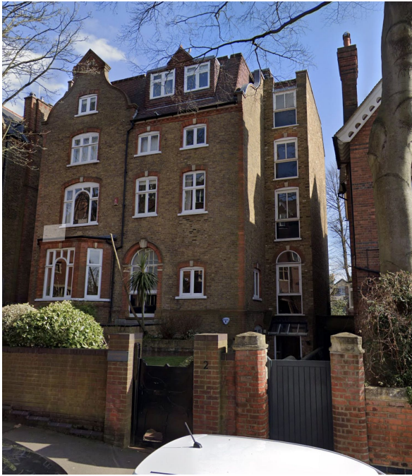
2 2 Holford Road, from the highway
