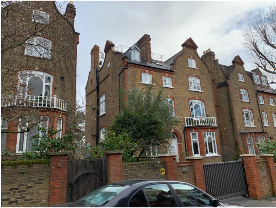
1 3 Holford Road, from the highway
