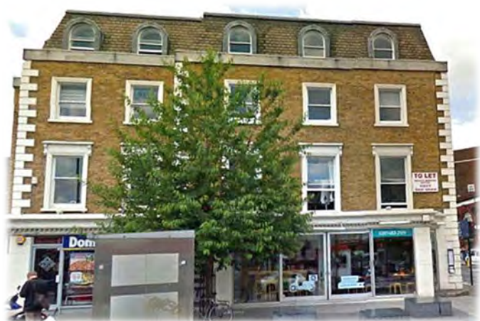
FRONT ELEVATION OF NOS. 155 – 157 REGENT'S PARK ROAD, 21 ST CENTURY
