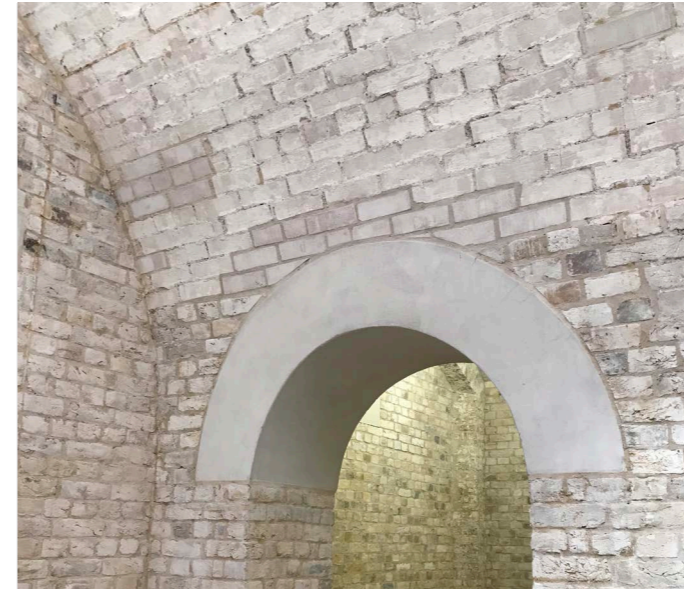
Light pre- cast stone / concrete arched lintel
