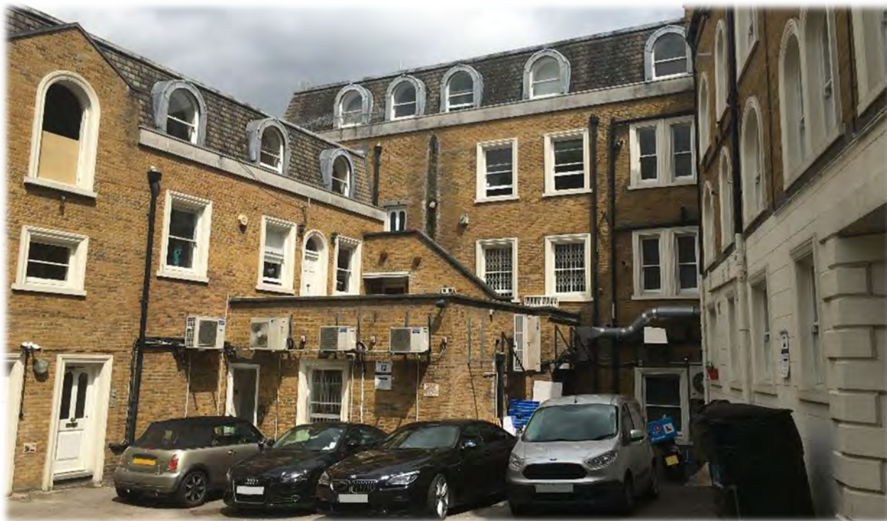
REAR VIEW OF THE SITE
