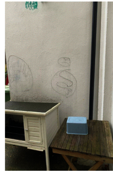
Image 13: Existing wall where proposed WC window to be reintroduced.
