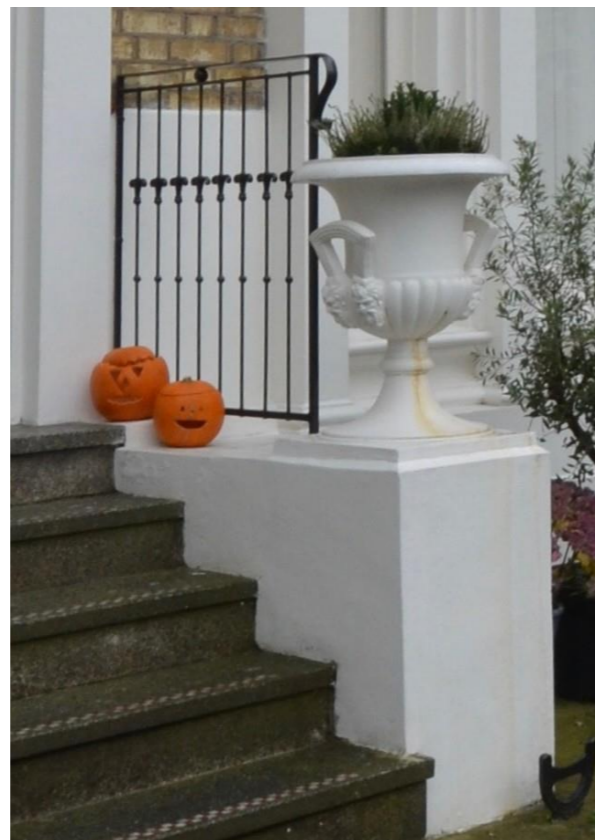
Image 7: The existing railings either side of the front door steps are to be replicated around the lightwell and to a proposed balcony to the rear. Existing terrazzo steps to be replaced with stone.
