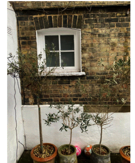
Image 14: Existing window at no.11
