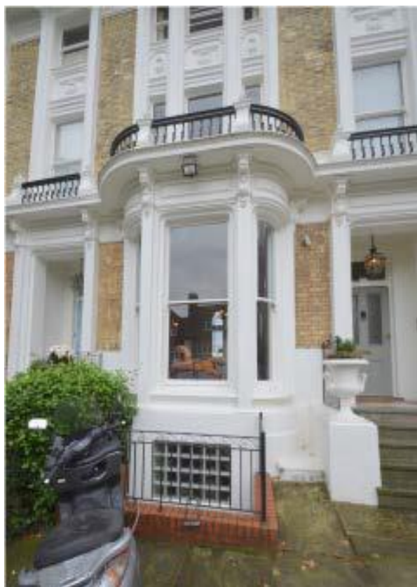
Image 6: Existing railings around the central lightwell to be replaced with railings to match the existing railings either side of the front door steps (see image 7) in finish, style, material and colour.
