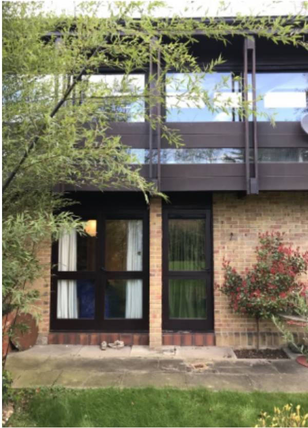
4. View of where the stairs will be
