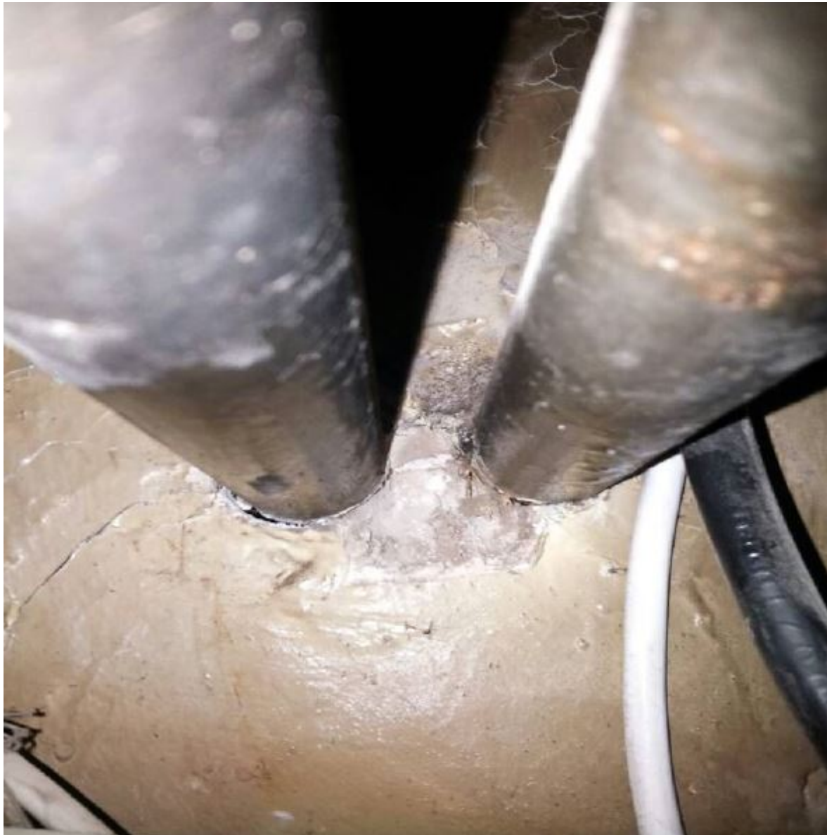
Figure 17: Extract from RPS Asbestos Survey Report 2017 – Photo of Pipes Penetrating Wall in Basement Level 1
