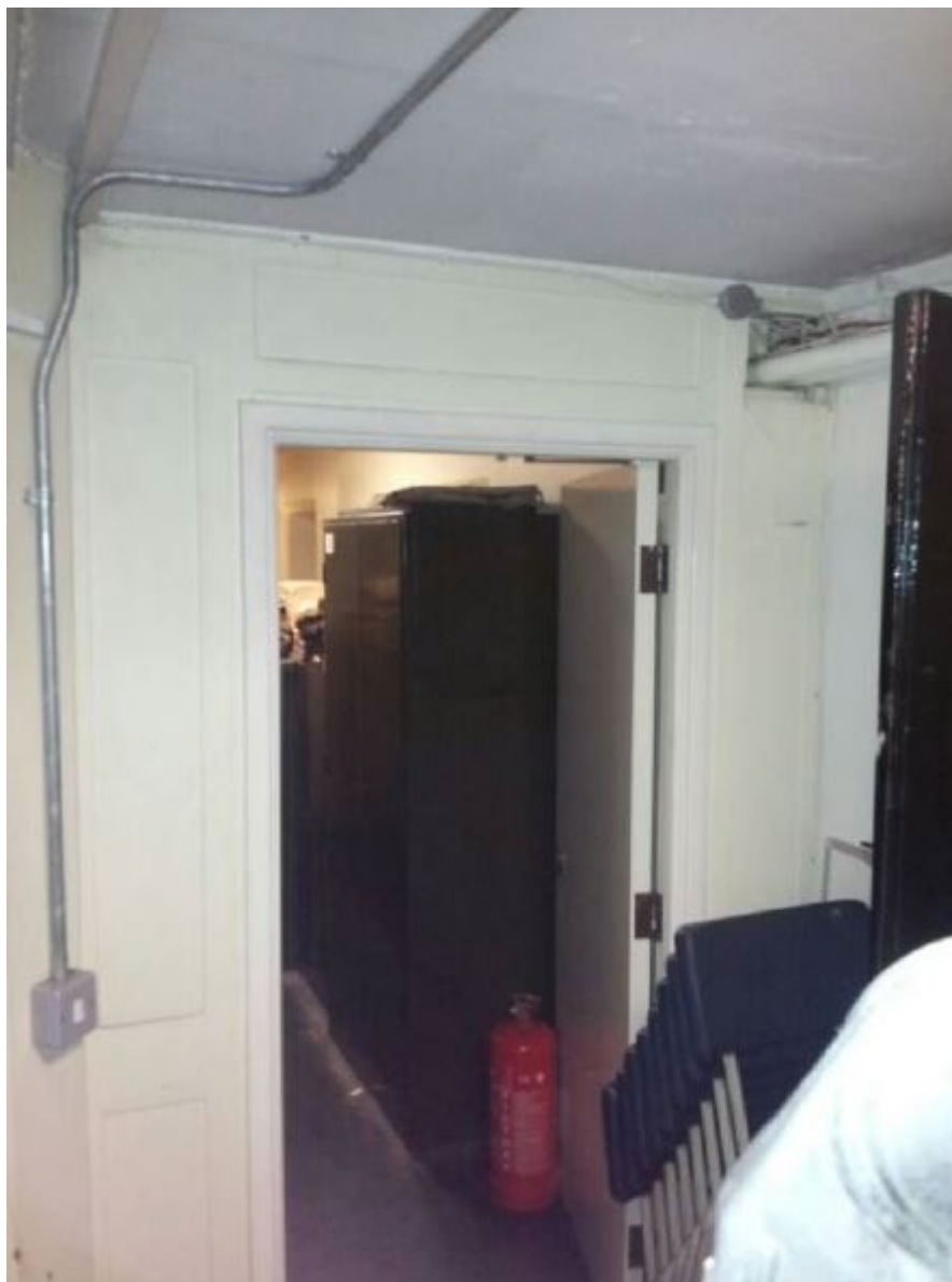
Figure 19: Extract from RPS Asbestos Survey Report 2017 – Photo of Insulation Boards around doorway on Ground Floor Level 2 Stair Lobby
