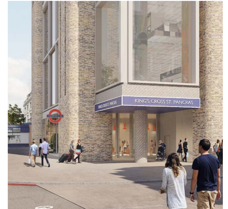
4 King's Cross Station Tube Entrance New step free access to King's Cross tube station, de cluttering the Euston Road
