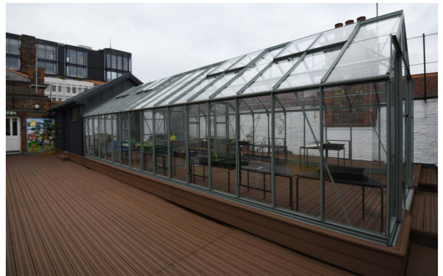
Argyle Primary School with its new roof biosphere funded by Precis
