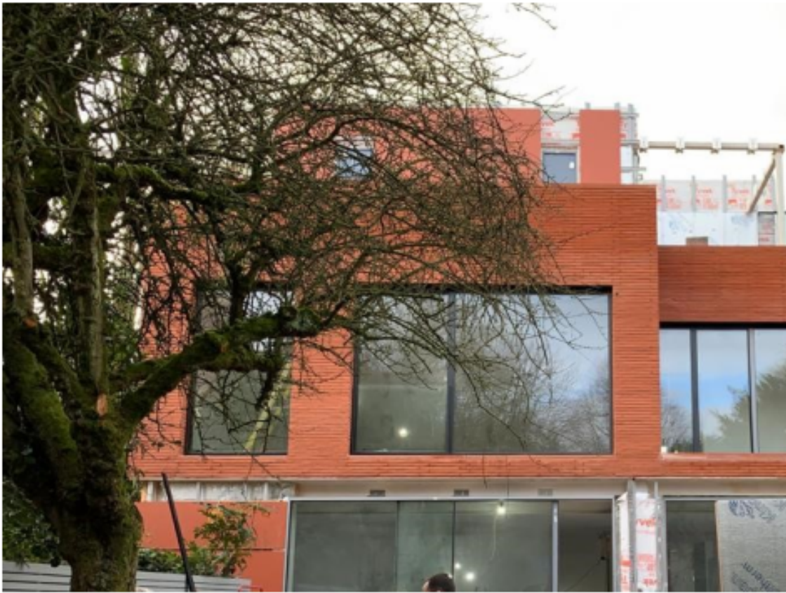
3. (above): View towards rear of 36 Redginton Road which is under construction
