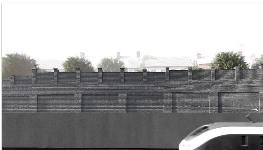
Figure 15 Illustration demonstrating proposed dark concrete finish for the proposed PVE Wall Berm, Parapet and Upstand Support Structure
