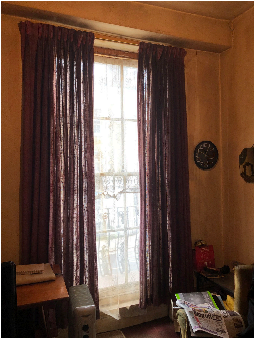
Figure 8: Internal view of window at first floor level
