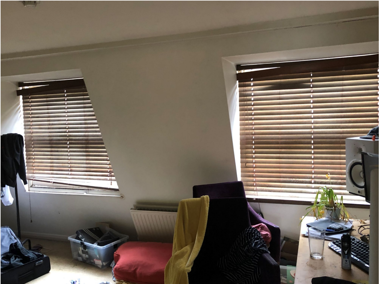
Figure 10: Internal view of windows at third floor level
