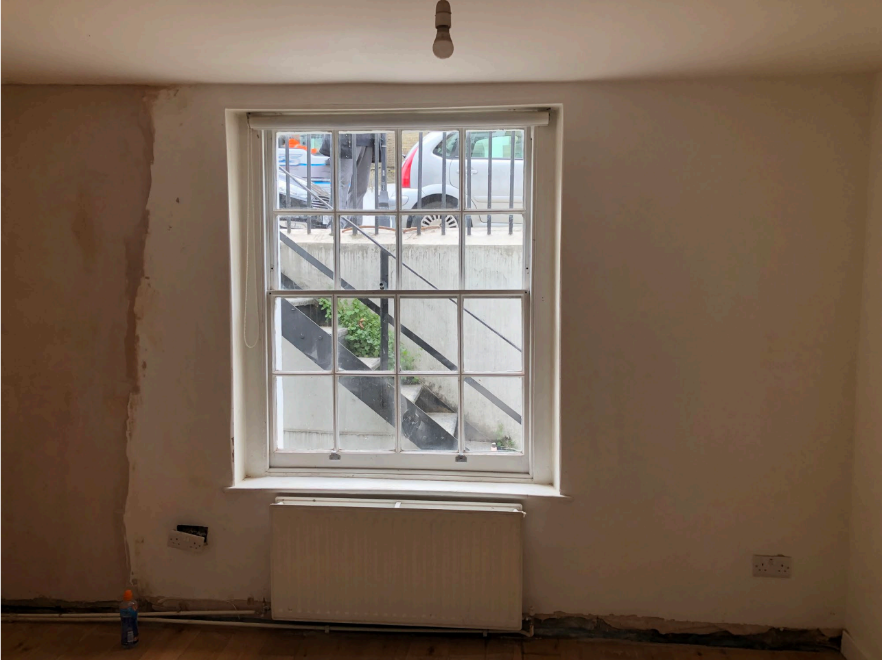
Figure 6: Internal view of window at basement floor
