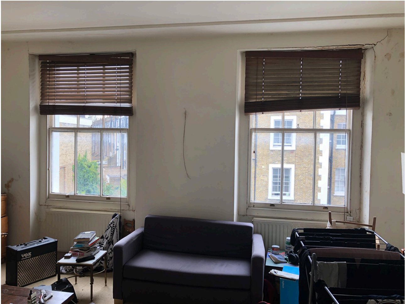
Figure 9: Internal view of windows at second floor level
