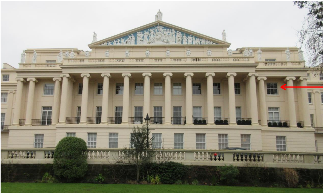
Figure 12: The front (west) elevation of the central block of Cumberland Terrace – the four southern windows (right) of the second floor comprise the subject site.
