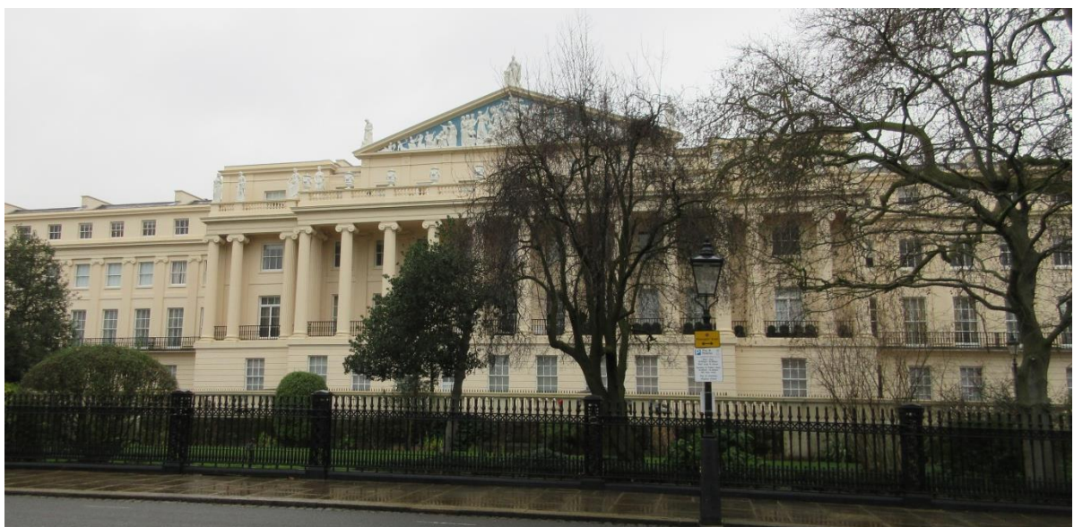
Figure 3: The subject site forms part of the grand architectural composition of the Grade I listed Cumberland Terrace from the Outer Circle.
