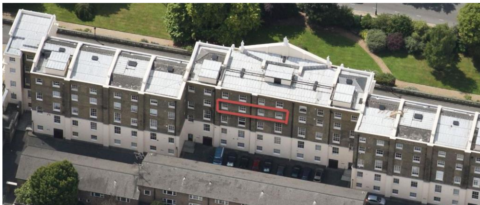
Overhead view 33 Cumberland Terrace Back Façade
