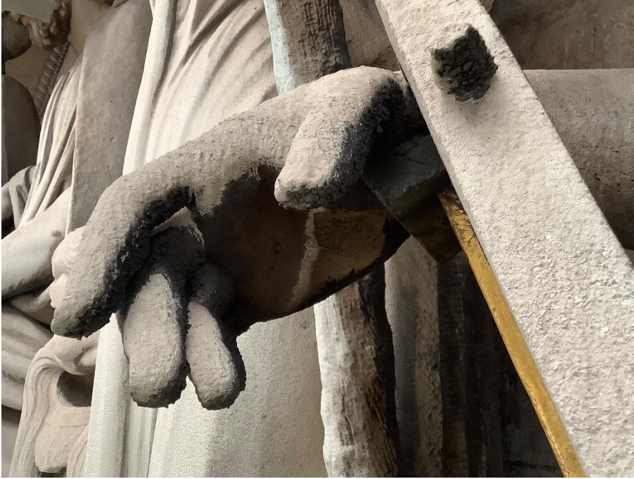
Image 4: Hand after partial laser cleaning showing removal of black gypsum crusts and no damage to underlying stone
