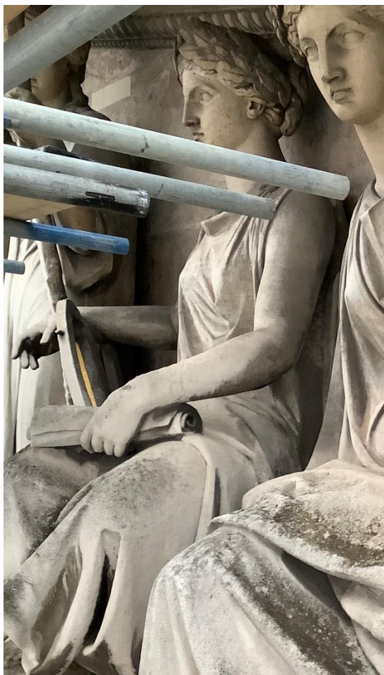
Image 1: Overall figure before tests, which also shows her proper left arm before cleaning off lighter black accretions with the laser
