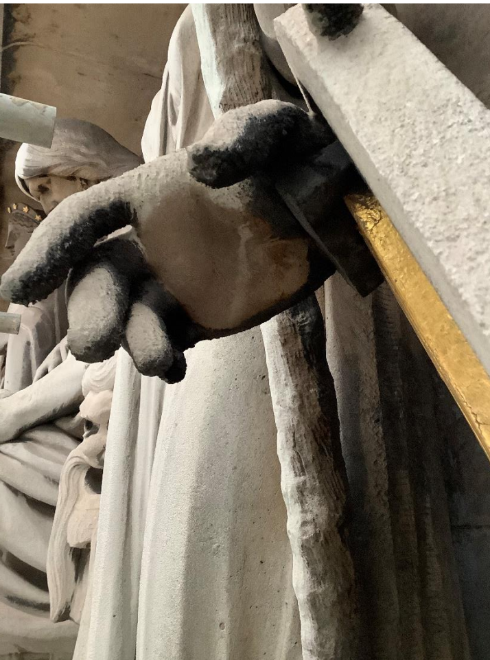
Image 4: Hand after partial laser cleaning showing removal of black gypsum crusts and no damage to underlying stone
