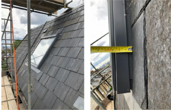
Close Up - Installed AOV and projection (80mm) from roof
