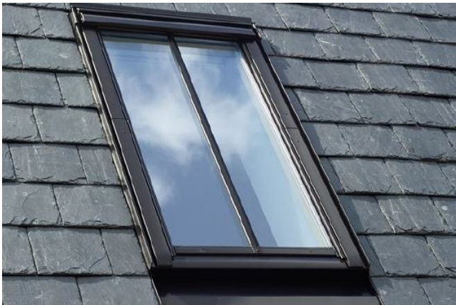
Fig. 4. Example of Conservation Style Roof light
