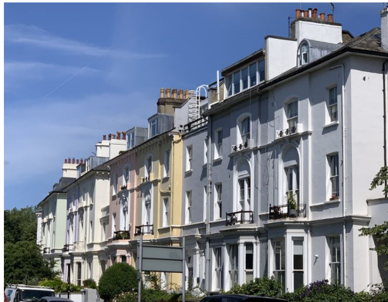
Fig. 3. Regent's Park Road Properties and Front roof alterations
