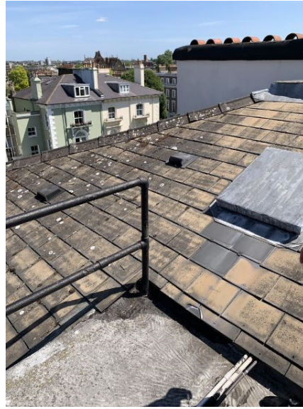
Fig. 2. Roof. Access hatch and metal balustrade
