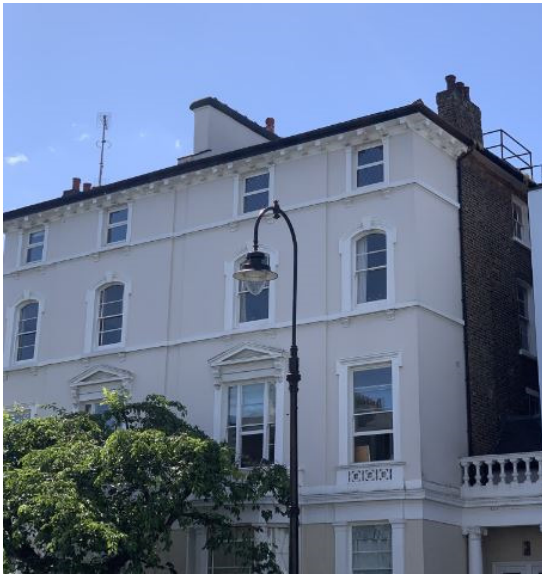
Fig. 1. Side elevation and metal balustrade
