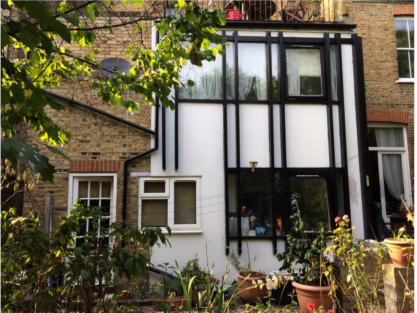
Existing rear elevation to Flat 1, 69 Greencroft Gardens showing the existing 2 storey outrigger extension and original tall patio doors to the right of the image. The roof of the outrigger forms an accessible terrace for the first floor flat above the subject property with metal railings to the usable area.
