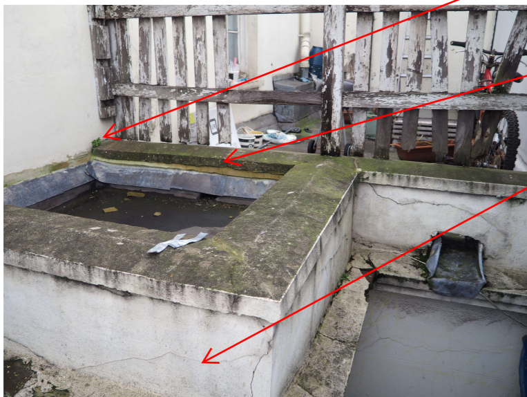
PHOTO 3: ROOF OF FRONT PORTICO
