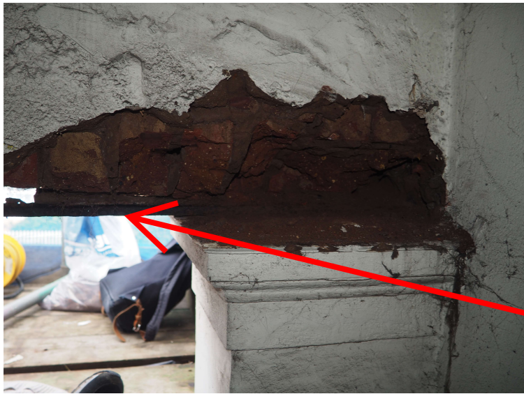
PHOTO 1: STEEL PLATE SUPPORTING PORTICO
