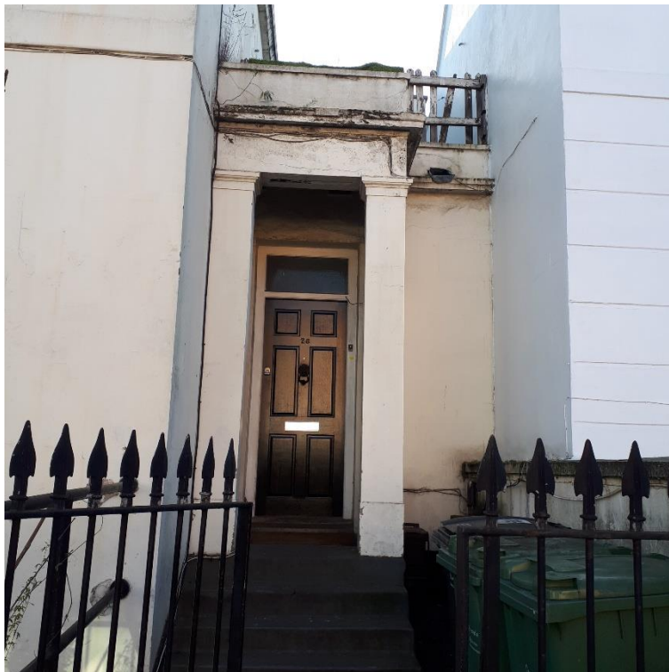
Plate 3a & 3b: Front Portico (Provided by Wates – surveyors)
