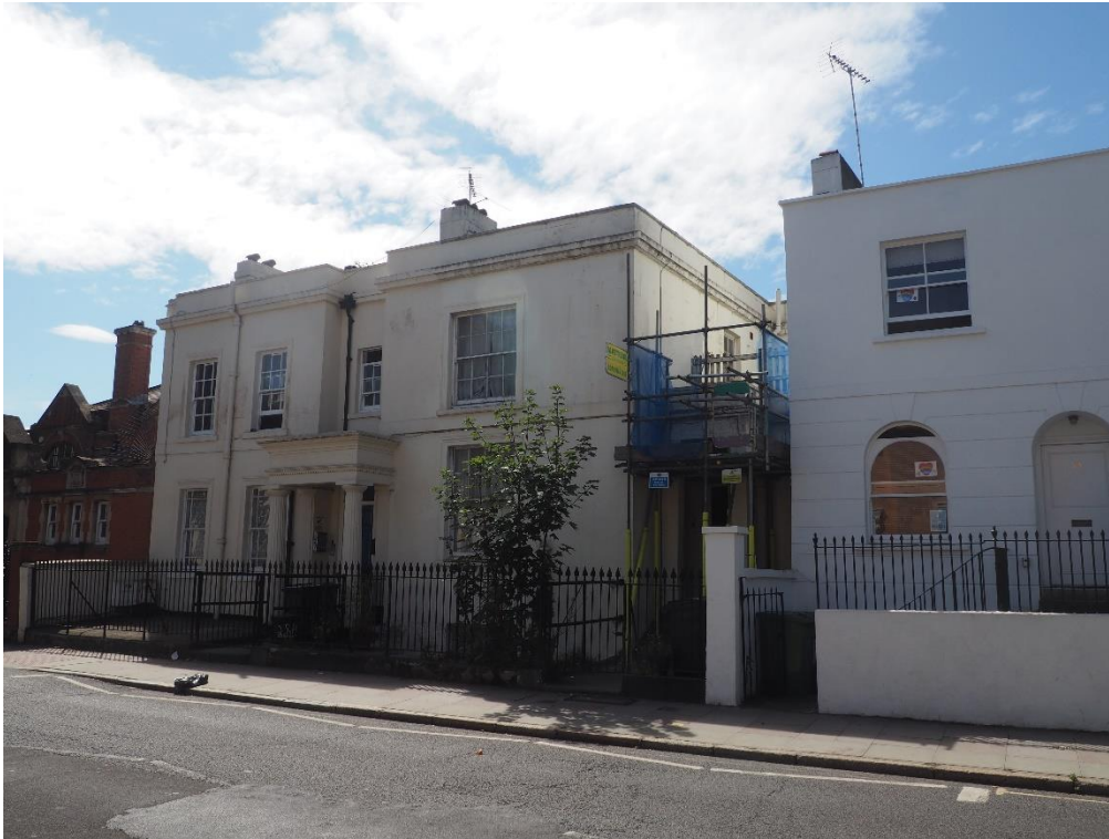
Plate 1: Front Elevation (Photo taken 13 th July 2020)
