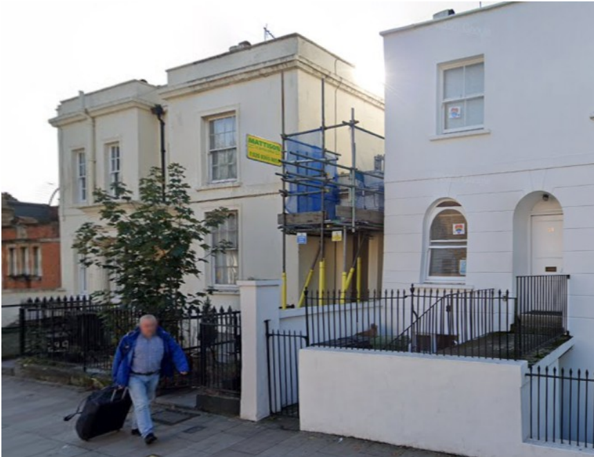
View towards no. 26 showing crash deck scaffolding in place
