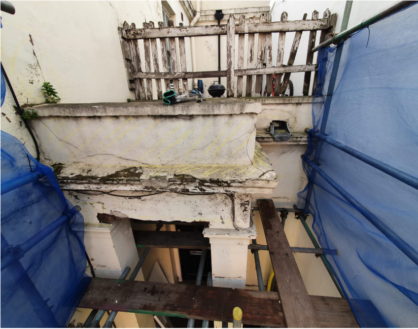
Front view of porch parapet showing concrete coping
