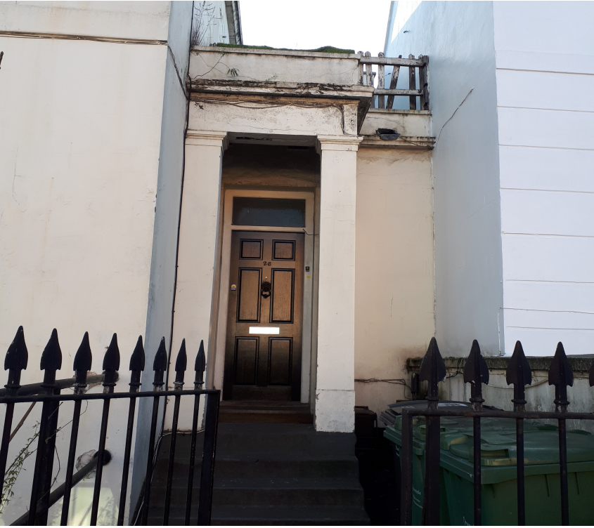
Porch of 26 Leighton Road before erection of crash deck
