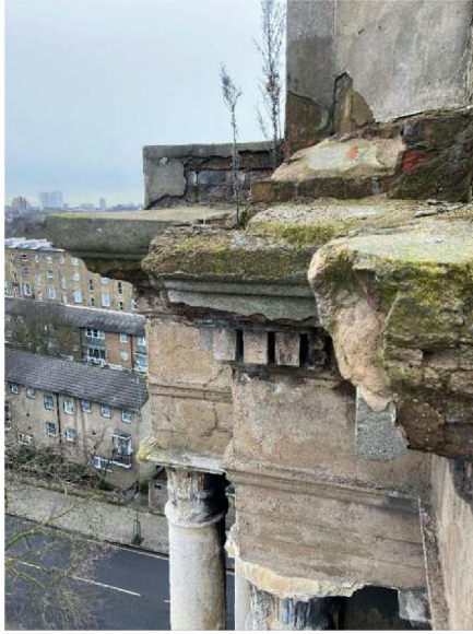
Img 09; failing render
