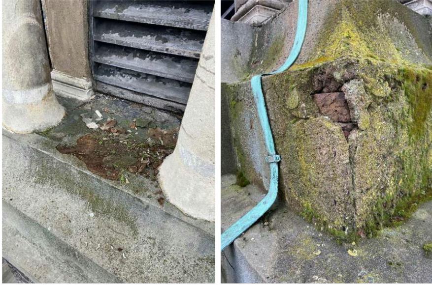
Img 13 and 14; debris and failing render exposing brickwork beneath
