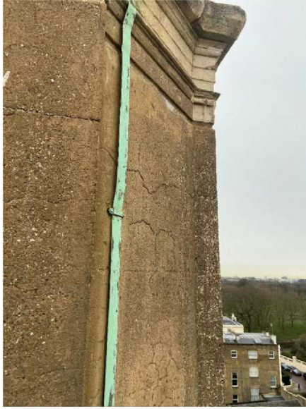
Img 01; cracked render
