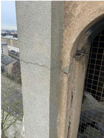
Img 03; cracking through render and repairs
