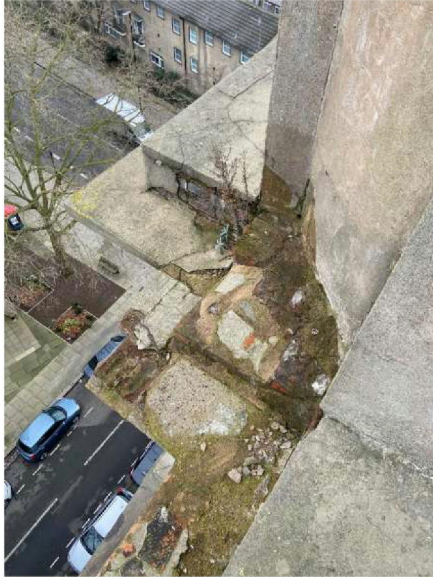
Img 05; failing render on sky-facing elements
