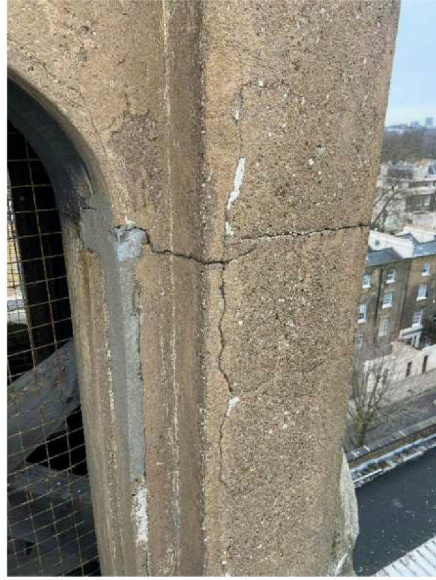
Img 02; cracked render and previous cement repairs
