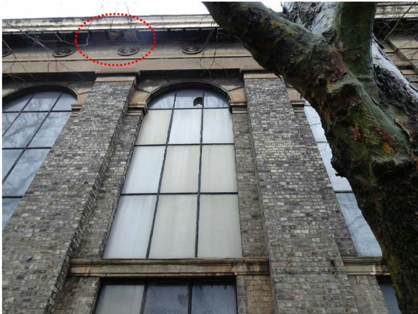
Img 19; rendered cornice on north elevation (liturgical) showing historic failure of rendered 'mutules' (circled)
