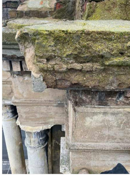
Img 10 and 11; failing render and brick dentils
