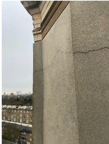
Img 04; horizontal cracking at high level.
