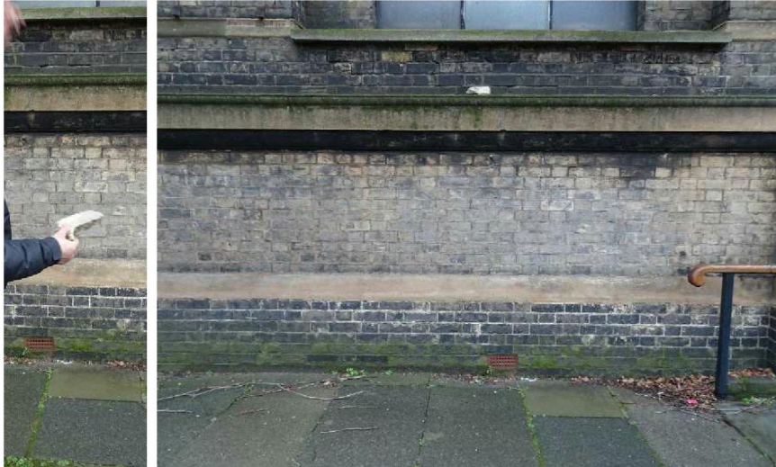
Img 17 and 18; render from debris found on the wall moulding which would have fallen in excess of 10m.
