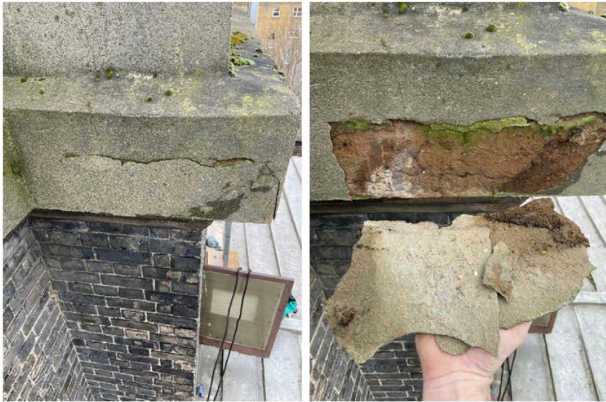
Img 15 and 16; cracked render failing when touched.
