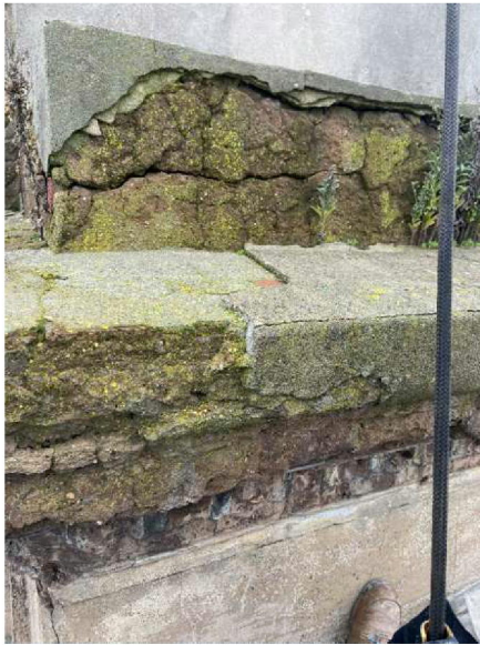
Img 09; failing render
