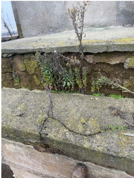
Img 07 and 08; failing render and plant growth. Note: steeplejacks have removed any plant growth on their recent visit)
