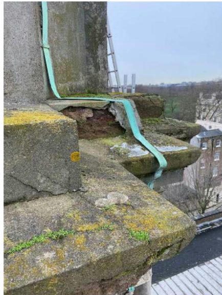
Img 07 and 08; failing render and plant growth. Note: steeplejacks have removed any plant growth on their recent visit)
