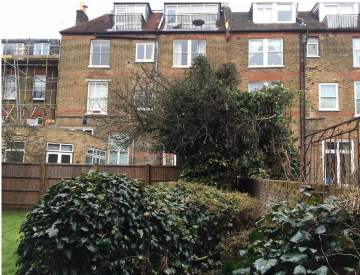
4. (Image above) Photograph of rear elevation with existing extension
