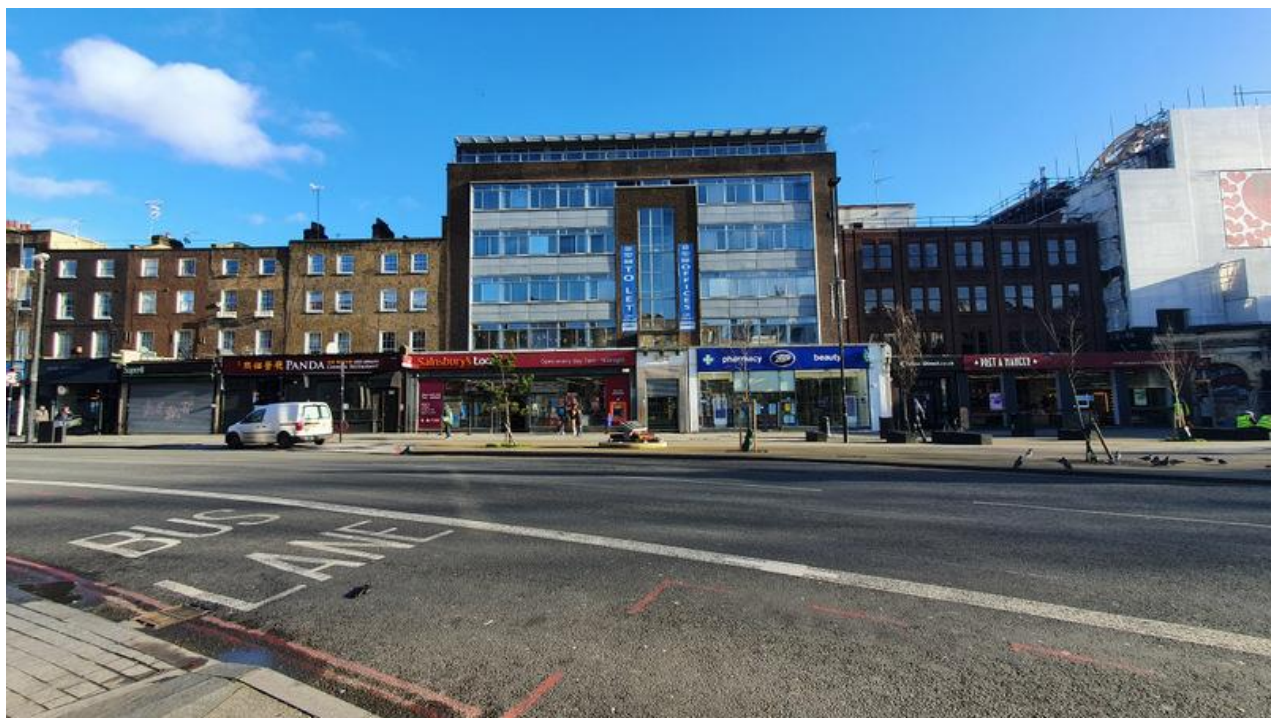
Below: Views across Camden High Street, looking east, with the 1960's building forming Nos8-12 rising above the c1790 terrace to the north. The scaffold-encased Camden Palace can be seen on the right.
