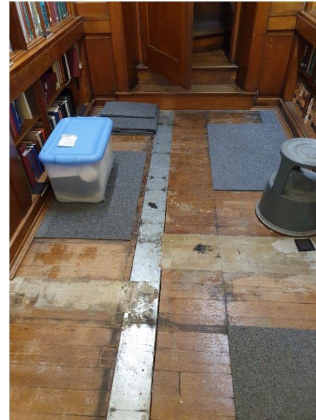
Examples of the metal cable boxing cutting through the floor
