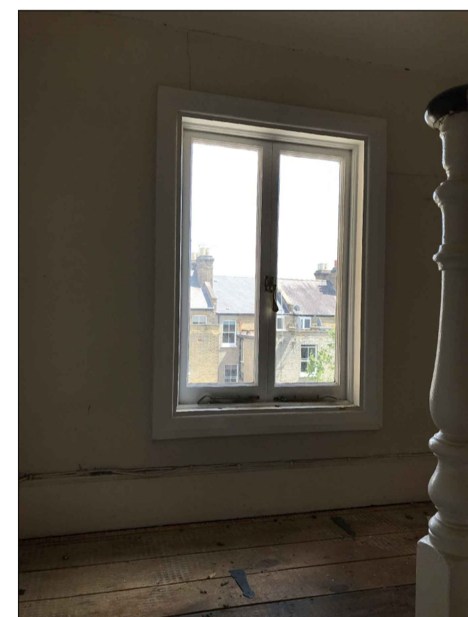
Typical Existing Casement Window
