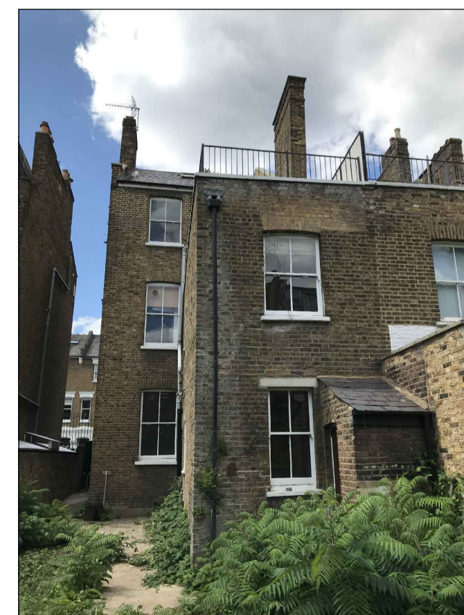
Typical Existing Sash Window
