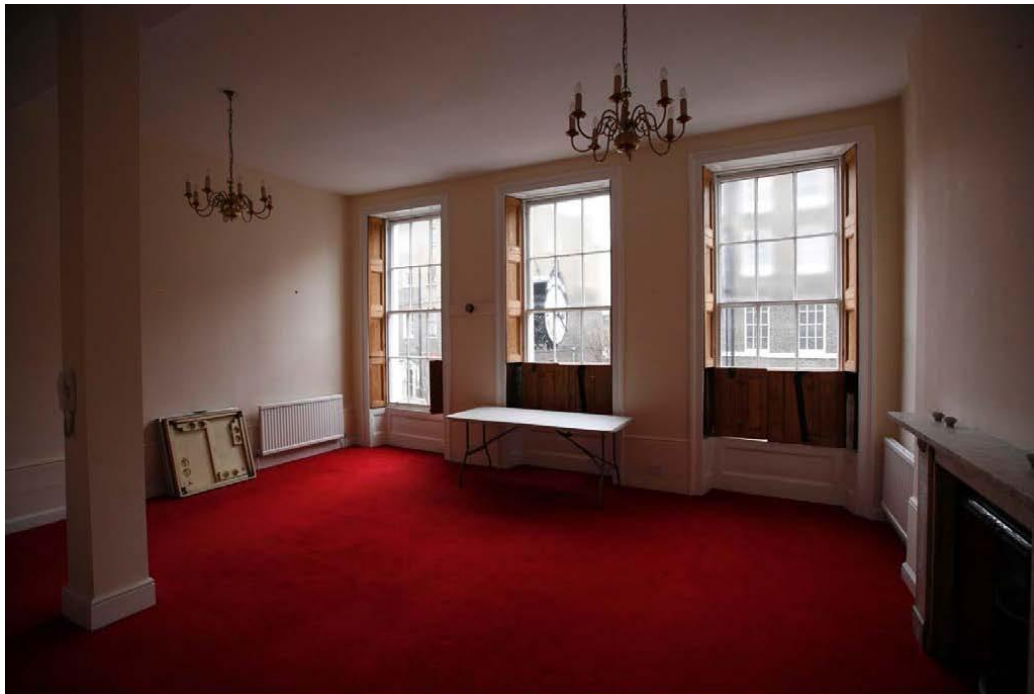
Image 23: A view towards the window of the front room at first floor level showing the non original column on the left which proves so detrimental to the original Georgian characteristics of the room. In addition, the non original clock can be seen through the central window.
