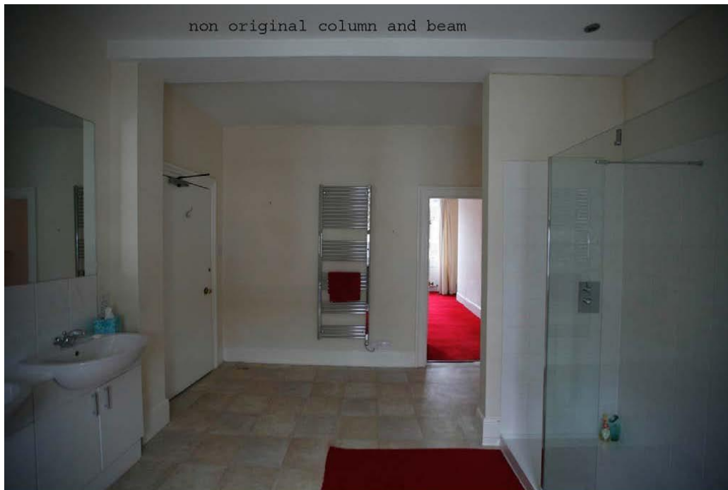
Image 27: A view of the non original bathroom at second floor level showing the non original columns and beam which are integrated in the current design proposal.
