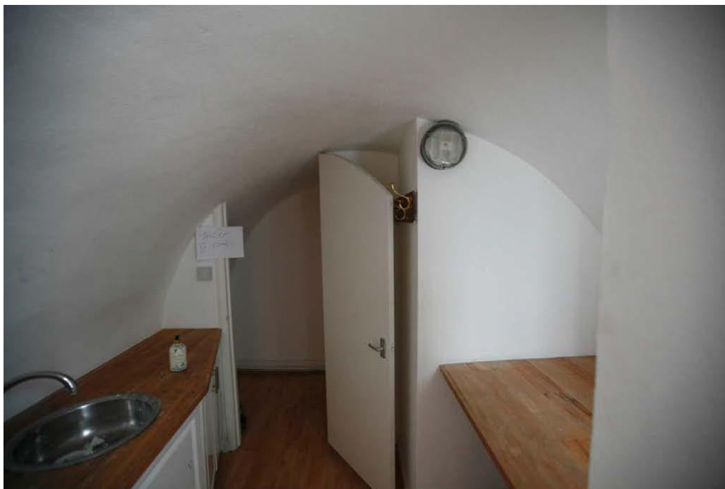
Image 14: The arched passage to the front area of the basement below the pavement, accommodating a non original kitchen area.
