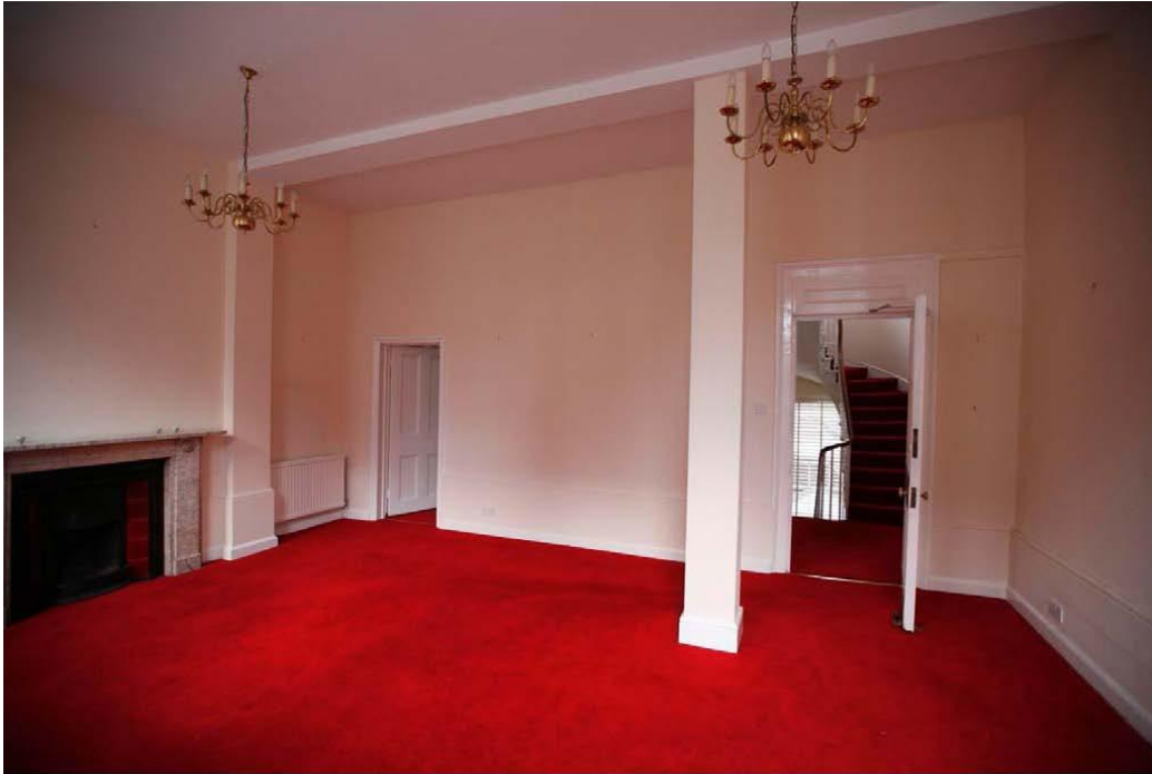
Image 19: Non original structural columns and beam as viewed at first floor level.
