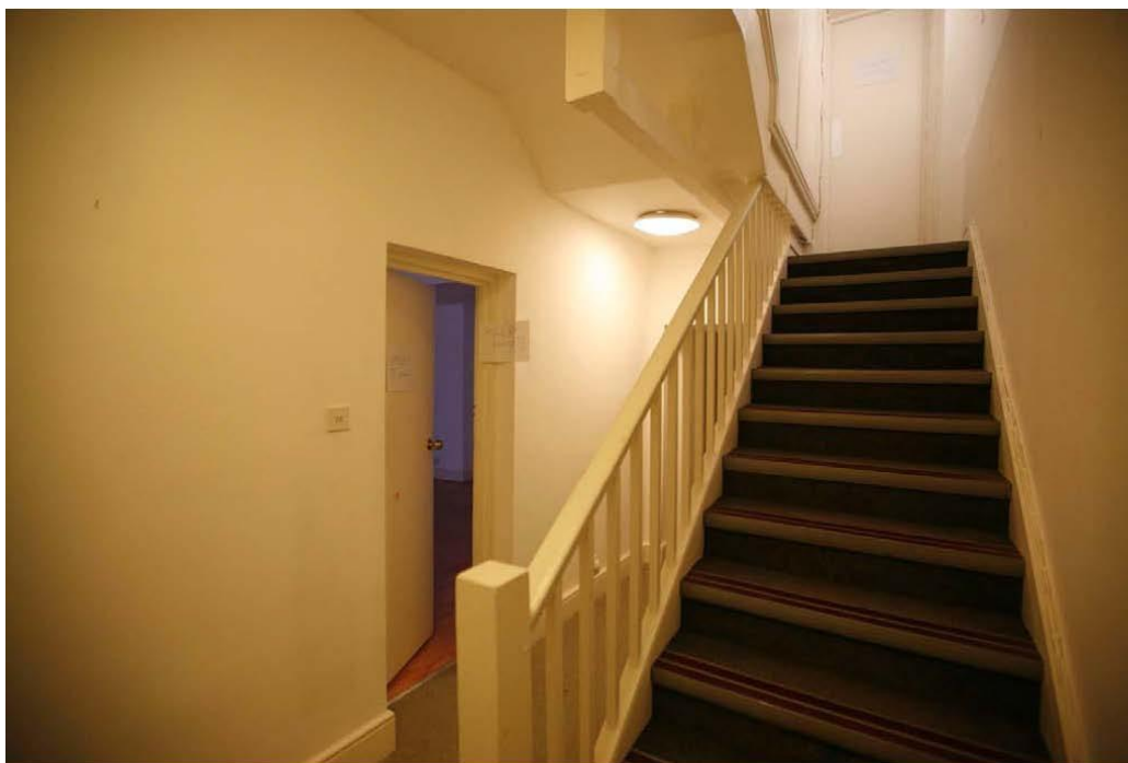
Image 15: Basement staircase enclosure: non original stairs from ground floor; exposed ducts; non original doors; out-of-character ceiling mounted light.
