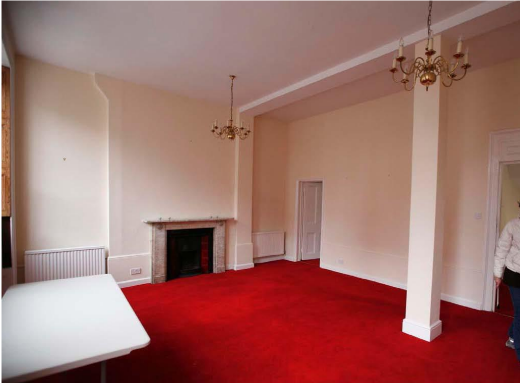
Image 24: The original marble fire place at front room of first floor level and non original column in wall.
