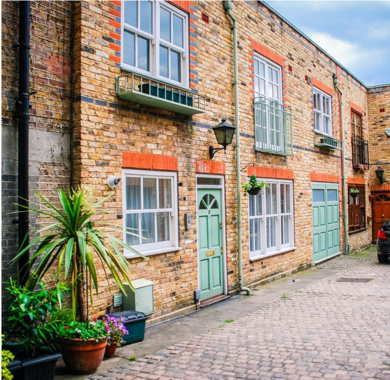
Photo of Existing Front Elevation
