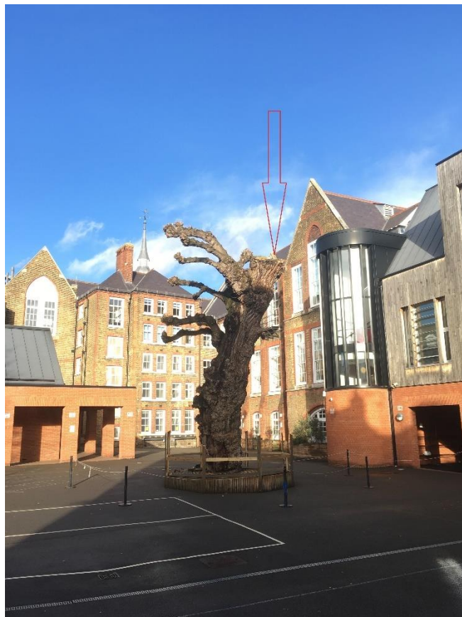
T1 viewed from a southerly direction with the location of the cavity indicated by the red arrow.
