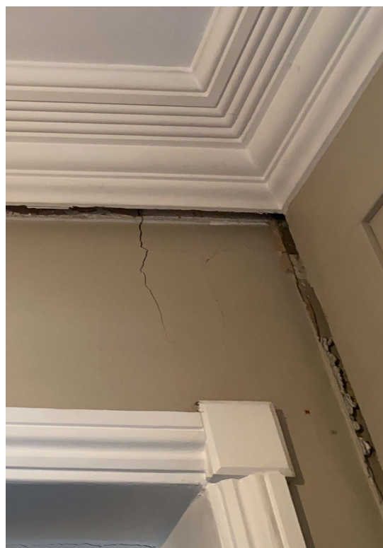
Internal cracking between portico and house
