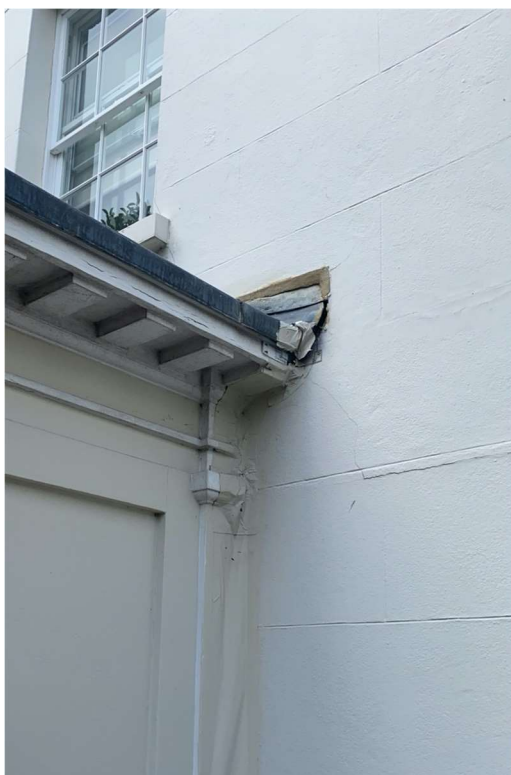
Widening gap covered with flashing tape
