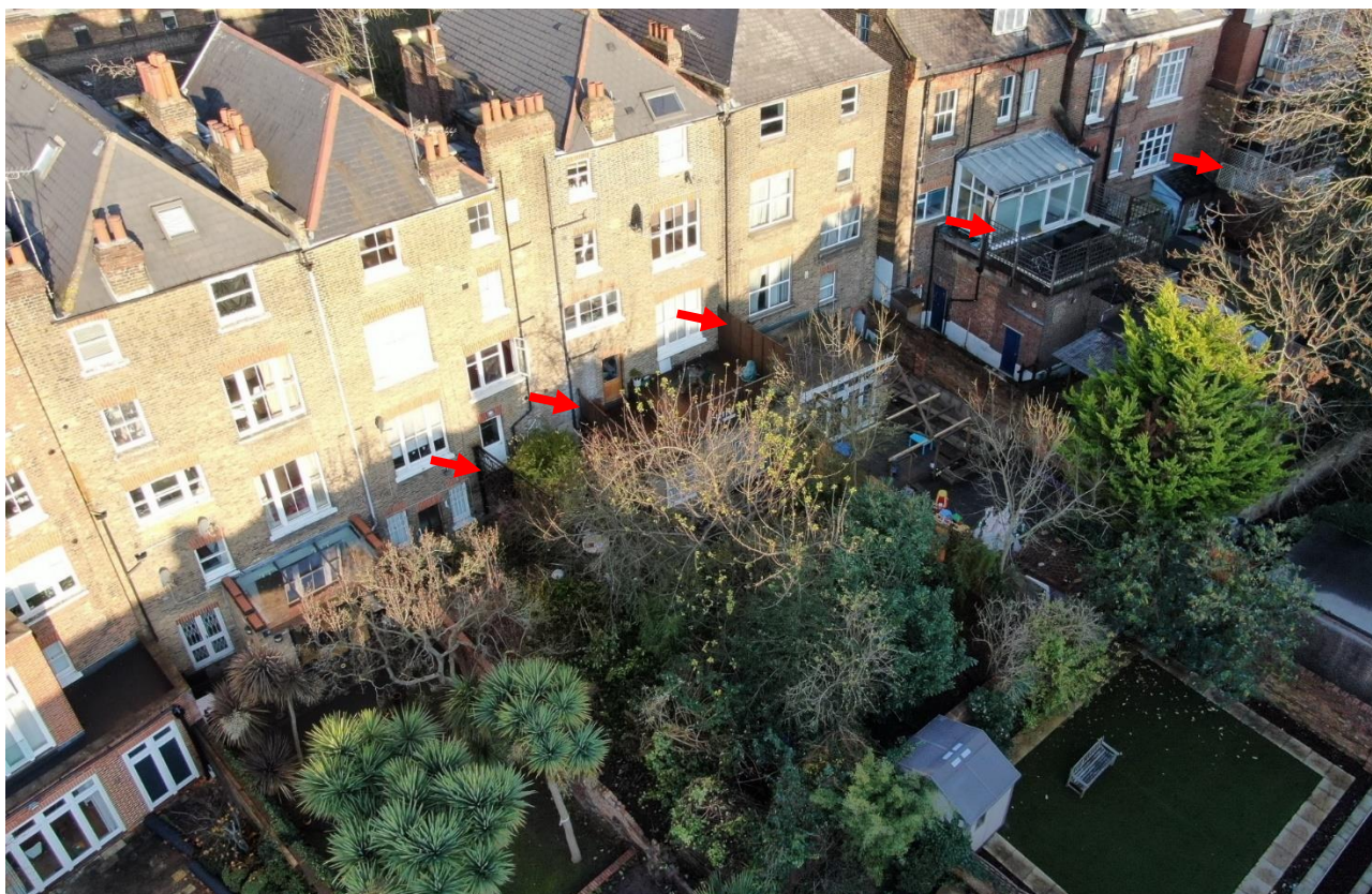
Photo 2: A drone photo, annotated with red arrows showing timber railings above ground level at the rear of properties on Broadhurst Gardens.
