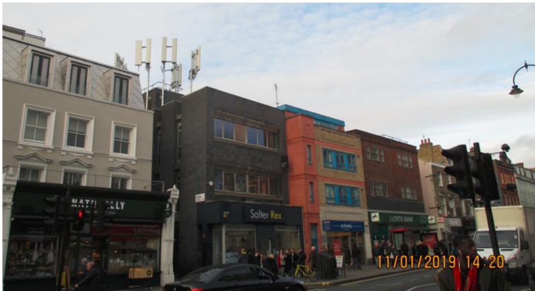
Unauthorised installation at 265-7 Kentish Town Road
