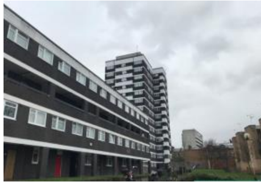
View from junction of Anglers Lane and Ragland Street
