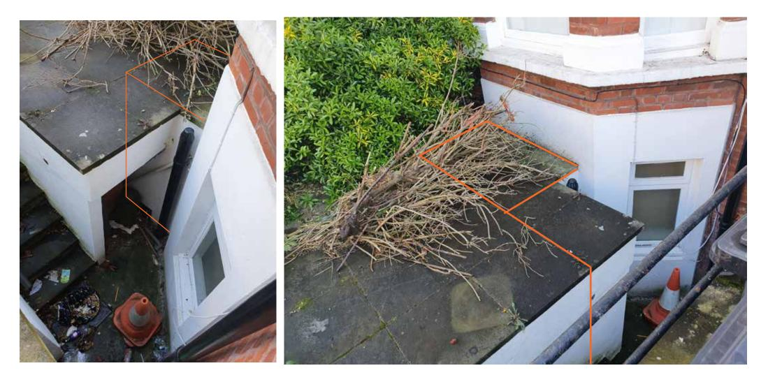
As can be seen on the above drawing it has partially been excavated already and used as a storage. The orange line shows the extent of excavation required. Possible 2 cubic meters only. This will improve living conditions in the bedroom.
