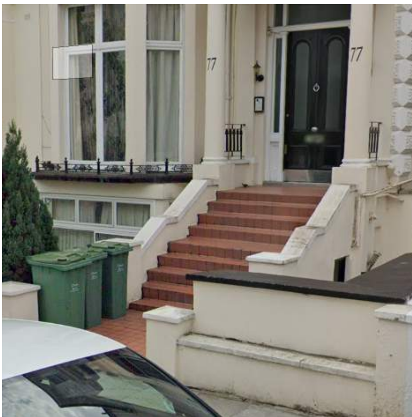
No 77- Lower ground floor, front window appears to be UPVC.
