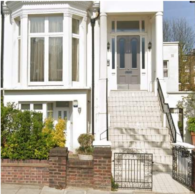
No 52- Lower ground floor door to front façade & timber windows.
