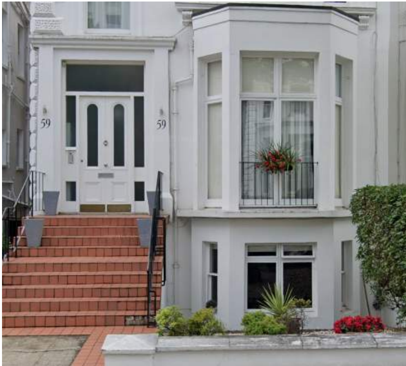
No 59- Lower ground floor top hung casement.
