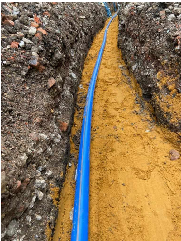
SITE PHOTO SHOWING BARRIER PIPE BEING INSTALLED
