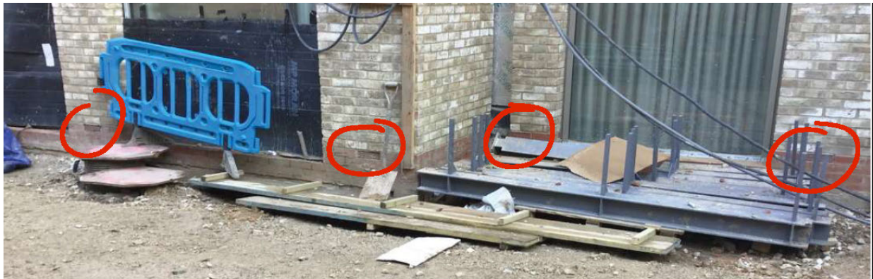
SUB-FLOOR VENTILATION POINTS
