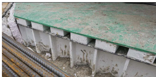
REINFORCED CAST IN SITU FLOOR SLAB
