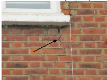
Cracking to front elevation
