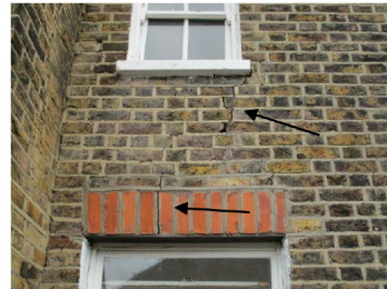
Cracking to rear elevation
