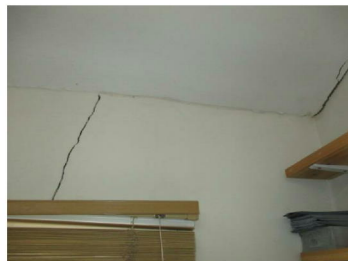
Cracking in flat d above rear window
