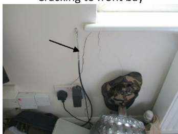
Cracking in flat D front bedroom
