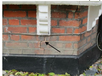
Cracking to front bay
