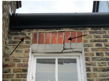
Cracking to rear elevation
