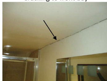
Cracking in flat D bathroom
