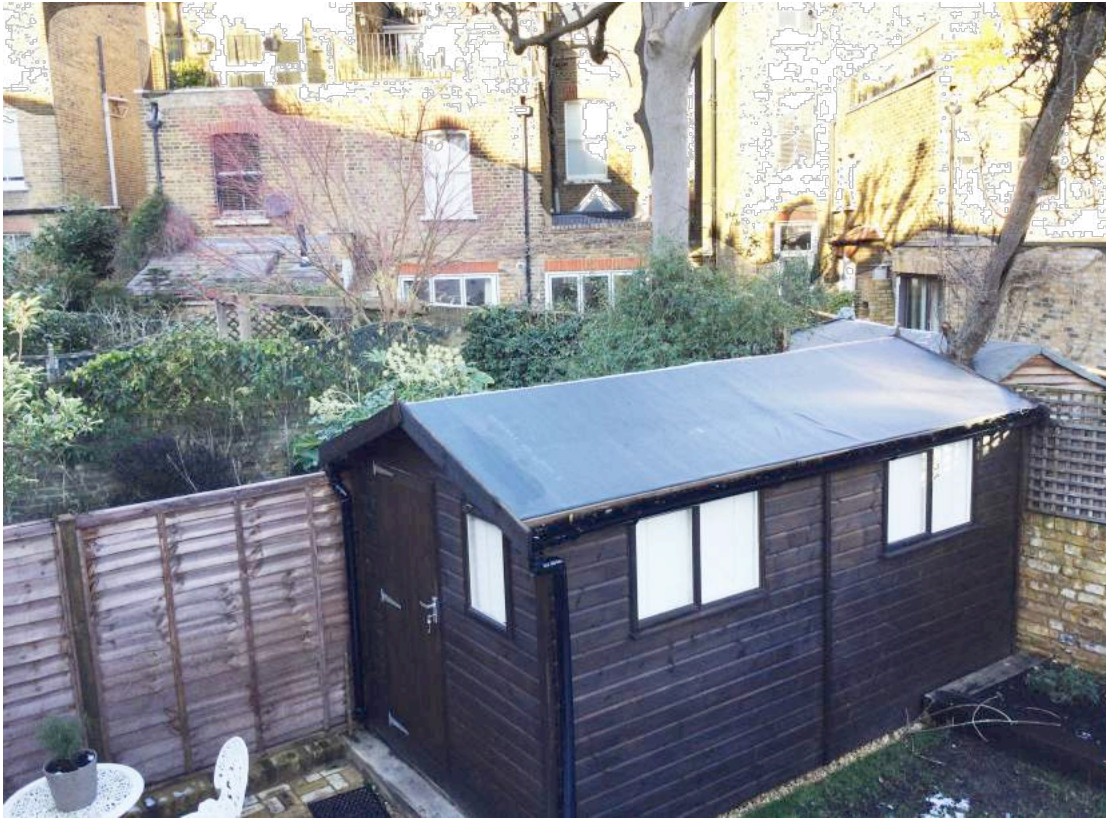
view of shed (as built)
