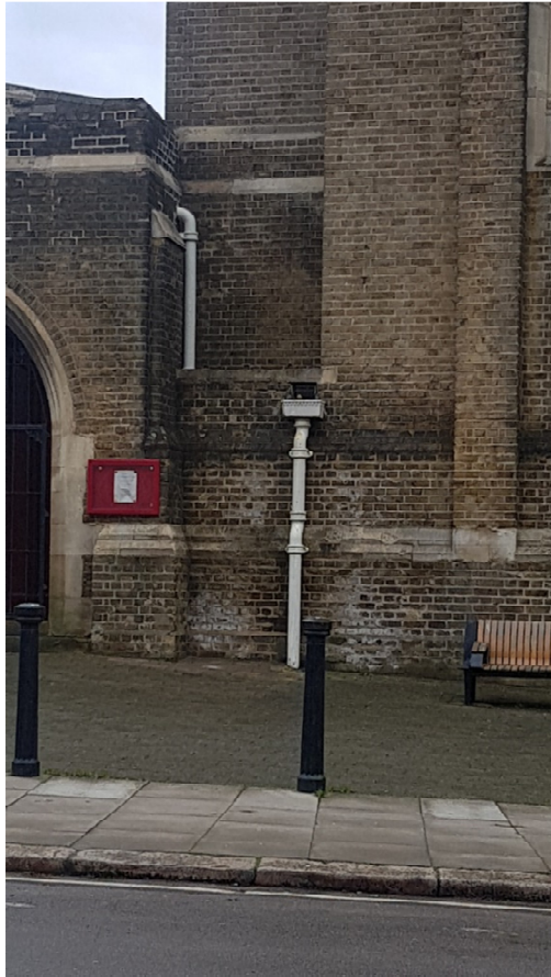
Pipes from the porch flat roofs snake through the ceiling and back out to discharge on one of Hare's 'secret gutters' where they exit to hopper heads.
