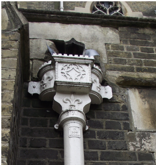
Sacristy hopper-head. It is proposed to place this on the visible south elevation where it will match the existing hopper-head and replace with the attached design from J and JW Longbottom Foundry.
