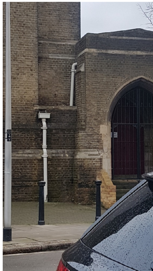
Pipes from the porch flat roofs snake through the ceiling and back out to discharge on one of Hare's 'secret gutters' where they exit to hopper heads.
