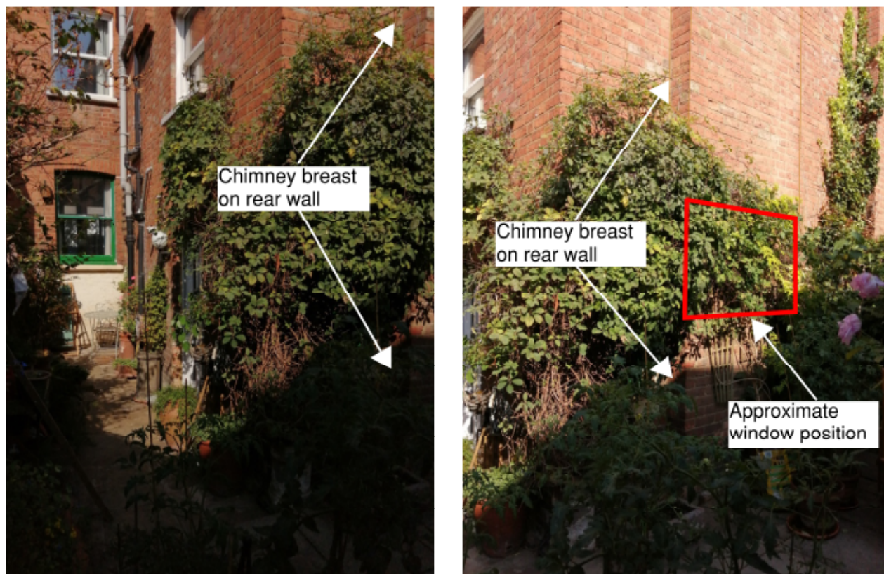
Photos 1 and 2 – showing the rear of the property and proposed window position within external chimney breast
